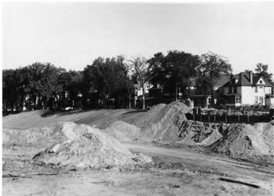
Demolition of homes for construction of I-94 through Rondo
