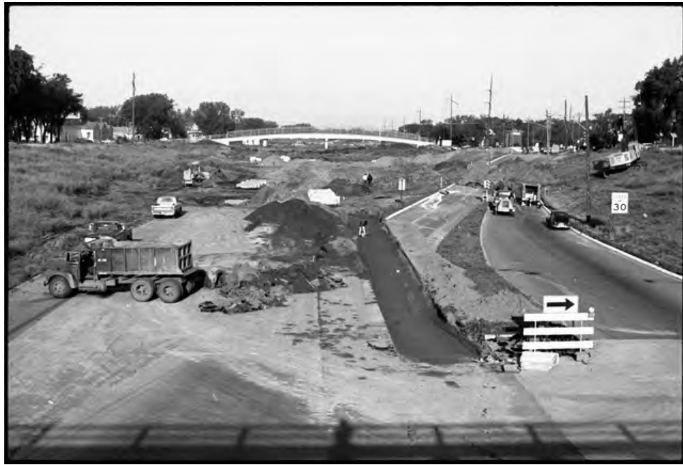
Demolition of homes for construction of I-94 through Rondo
