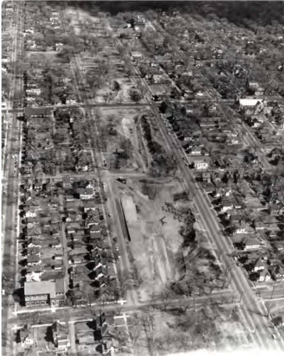
Demolition of homes for construction of I-94 through Rondo
