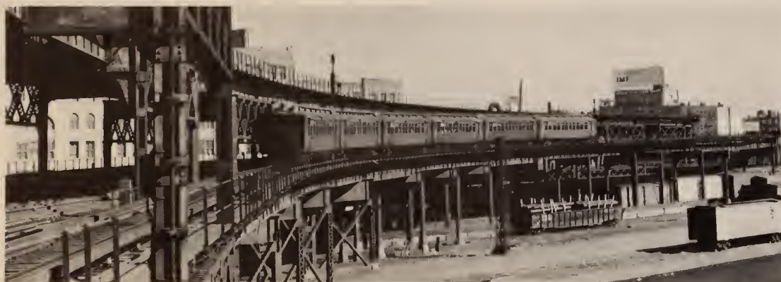
TOP: The bi-level swing bridge that carried Second and Third Avenue el trains across the Harlem River between Manhattan and The Bronx. In this view looking westward in 1940 a 5-car train of gate cars is Manhattan-bound in the morning rush hour. George E. Votava. MIDDLE LEFT: An uptown train of MUDCs comes off the lower level of the bridge and crosses over the New Haven Railroad yards in March 1954. Herbert H. Harwood. LOWER LEFT: A view of the Harlem River crossing from the electrified New Haven Railroad tracks in 1940. A deadheading train of Composite cars heading for The Bronx on the upper level and an uptown MUDC local below pass during the morning rush hour. George E. Votava. LOWER RIGHT: An uptown train of MUDCs leaves 129th Street and approaches the Harlem River Bridge in 1954. Herbert H. Harwood
