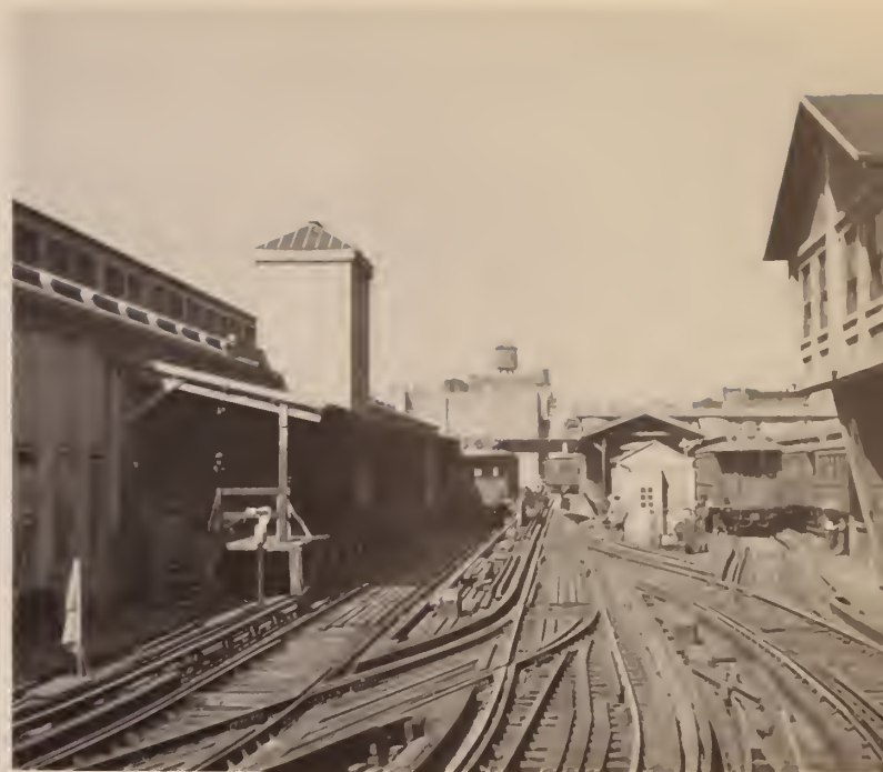
Votava. BOTTOM: A view of 129th Street in 1949, showing the express track bypassing the station at right and the overhead walkway connecting the platforms. David L. Klepper
