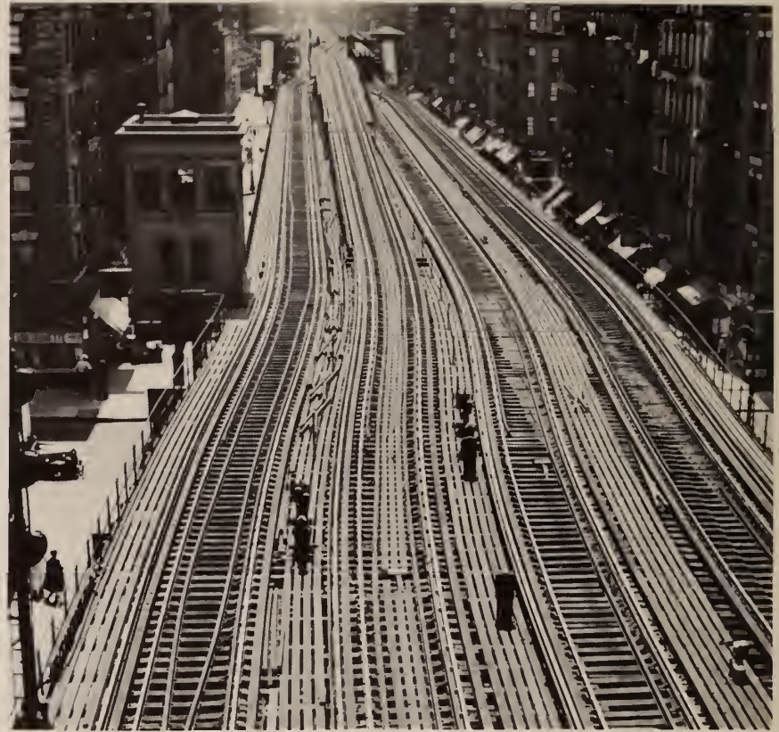
A highway of wood and steel! This view of the Ninth Avenue el looking south over Eighth Avenue from the 151st Street station illustrates the typical Manhattan elevated roadbed, where wooden ties and wooden walkways predominated. The three-track right-of-way branched into four with a flying junction to separate trains terminating at 155th Street from those routed to and from The Bronx.
