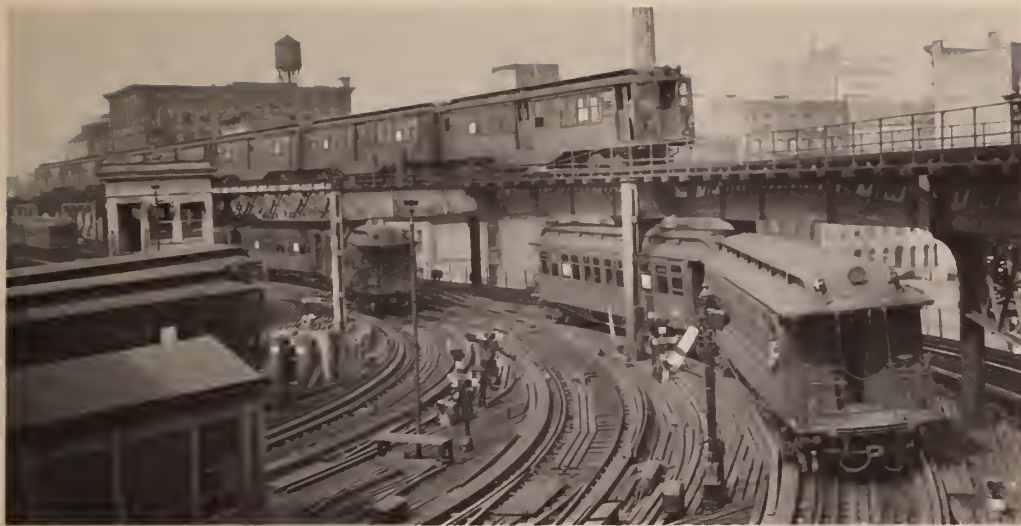
The 129th Street terminal and yard complex was built between 1886 and 1898 to serve both the Second and Third Avenue els as well as the Suburban line to The Bronx. The station was used to turn back local trains on both lines and thus served as a transfer point. UPPER LEFT: A view of the curve at Third Avenue and 129th Street in June 1940. A northbound train of Composites bound for The Bronx zips by the station and several trains of gate cars. George E. Votava. UPPER RIGHT: Looking west at the 129th Street terminal from Second Avenue. The platform at left was part of the yard and not open to passengers. George E.
