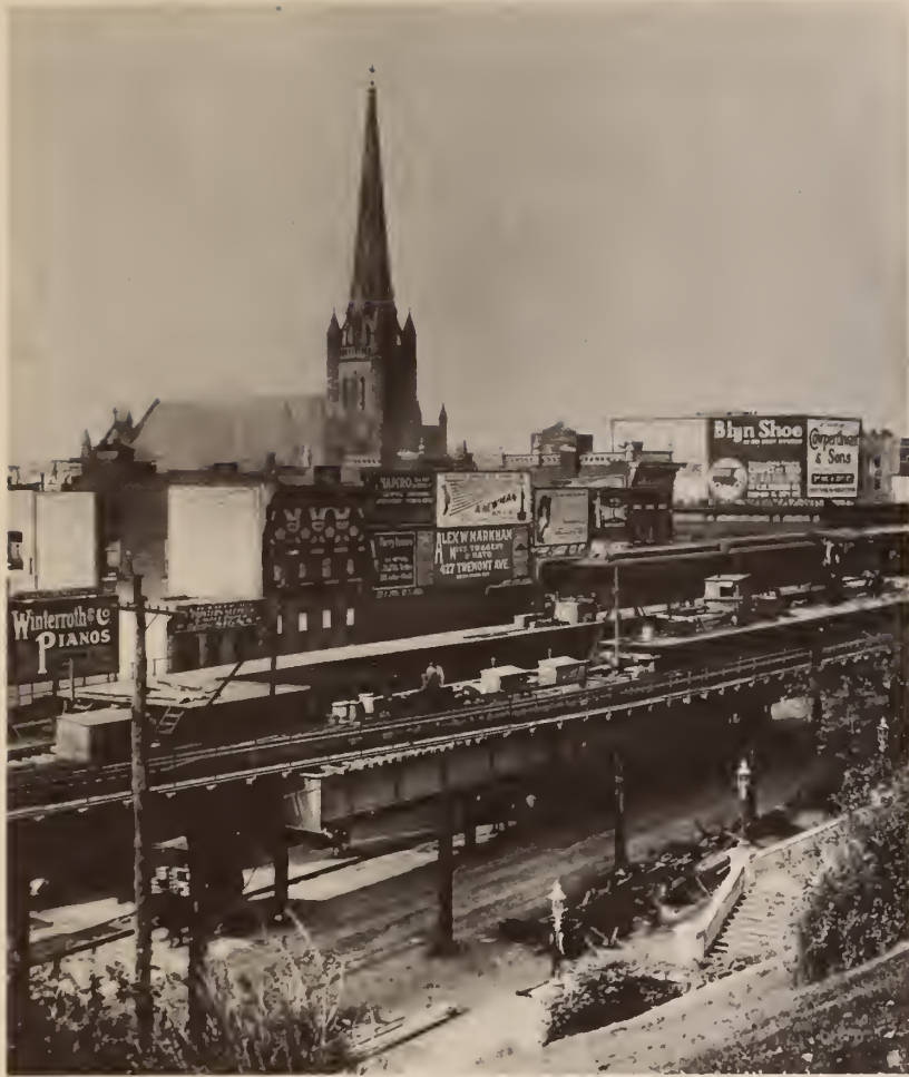
UPPER LEFT: The central Bronx developed rapidly after through service from Manhattan was inaugurated at the end of the nineteenth century. As part of the Dual Contracts a third track was added to the Third Avenue el through both Manhattan and The Bronx. In October 1915 the work of rebuilding the Tremont Avenue station of the "Suburban" into an express stop was nearing completion. courtesy Francis J. Goldsmith, Jr. UPPER RIGHT: A grade separated junction between the Ninth Avenue el and the Jerome Avenue branch of the Lexington Avenue subway was constructed in the marshes of the West Bronx as part of the Dual Contracts. This 1918 view shows a subway shuttle train of Low-V cars laid up in the center track. Interborough Archives. LOWER RIGHT: By 1940 the neighborhood along River Avenue had been developed for many years. In this view from the end of the uptown platform, a downtown MUDC-equipped Ninth Avenue el train rolls into 167th Street. The sign in front of the workmen maintaining the signal indicated the stopping point for 10-car subway trains and 7-car (Manhattan) el trains.
