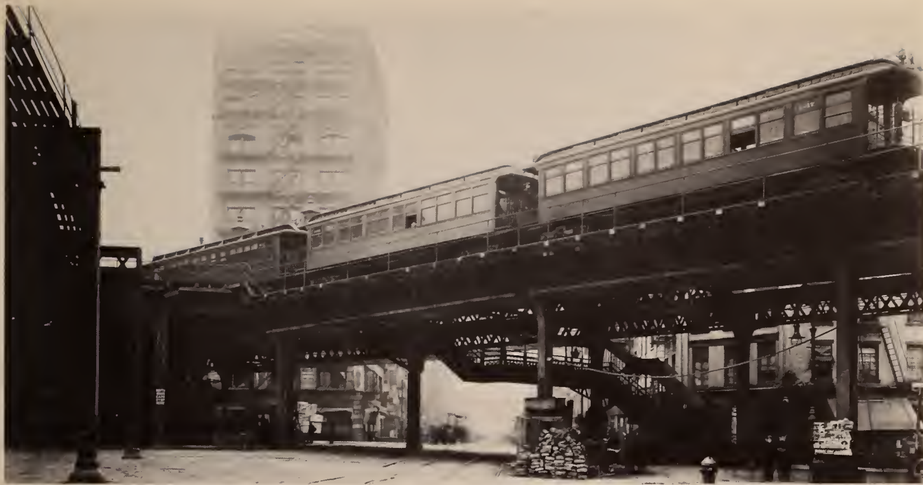
The Chatham Square-City Hall area of lower Manhattan was host to a huge complex of tracks in the sky. Flying and burrowing junctions permitted Second Avenue and Third Avenue el trains to reach either City Hall or South Ferry with a minimum of conflicting movements. TOP: Looking northeast along East Broadway at Chatham Square in 1916, during the reconstruction of the junction. A train of gate cars from Second or Third Avenue heads for South Ferry. Interborough Archives . LOWER LEFT: A Third Avenue express of Composites heads toward the lower level of the City Hall terminal in this view southwest along Park Row from Chatham Square in 1940. George E. Votava . LOWER RIGHT: Looking southward along the Bowery from the Canal Street station of the Third Avenue el showing the beginning of the Chatham Square junction. Note that access to the lower level (City Hall branch) and the upper level (South Ferry branch) from both the express and local tracks was without grade crossings. Herbert H. Harwood . Additional photos of the Chatham Square area are on the front and rear covers.
