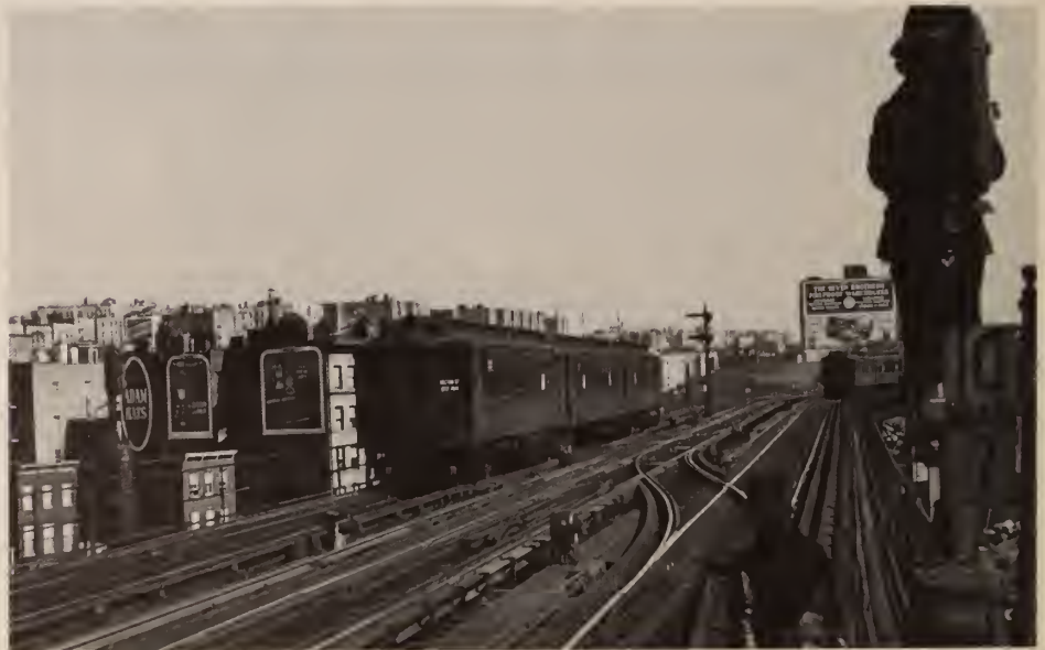
UPPER LEFT: The central Bronx developed rapidly after through service from Manhattan was inaugurated at the end of the nineteenth century. As part of the Dual Contracts a third track was added to the Third Avenue el through both Manhattan and The Bronx. In October 1915 the work of rebuilding the Tremont Avenue station of the "Suburban" into an express stop was nearing completion. courtesy Francis J. Goldsmith, Jr. UPPER RIGHT: A grade separated junction between the Ninth Avenue el and the Jerome Avenue branch of the Lexington Avenue subway was constructed in the marshes of the West Bronx as part of the Dual Contracts. This 1918 view shows a subway shuttle train of Low-V cars laid up in the center track. Interborough Archives. LOWER RIGHT: By 1940 the neighborhood along River Avenue had been developed for many years. In this view from the end of the uptown platform, a downtown MUDC-equipped Ninth Avenue el train rolls into 167th Street. The sign in front of the workmen maintaining the signal indicated the stopping point for 10-car subway trains and 7-car (Manhattan) el trains.
