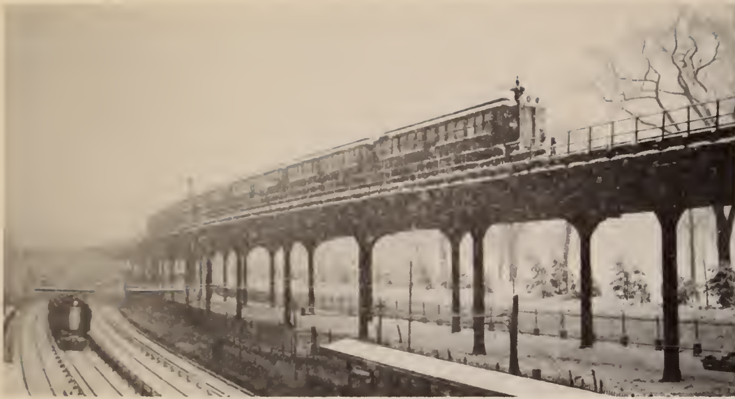
ABOVE: A snowy day in The Bronx. From Fordham Road to Bronx Park the Third Avenue el structure was built over private right-of-way between the New York Central tracks and the grounds of Fordham University. This 1938 view shows a train of Composites on the el and a train of New Haven Railroad MUs on the Harlem Division just beyond the Fordham station platform. E. Alfred Seibel. BELOW: The Third Avenue el at 180th Street station. An uptown train of MUDCs leaves the station and approaches a string of gate cars laid up on the express tracks. Robert L. Presbrey collection
